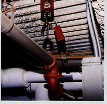
The clevis hanger in the center of the photograph fell apart and the rear hanger clevis is sufficiently displaced to have bent the ceiling bolt. There are chatter marks on the pipe in the front clevis, all indicating that this system went into resonance even though the accelerations were only 0.15gV and 0.2gH. Proper sway bracing, axial restraint and upper limit stops could have prevented this damage.
