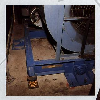
This large fan did not come down because there were control cables to prevent pendulum motion.
