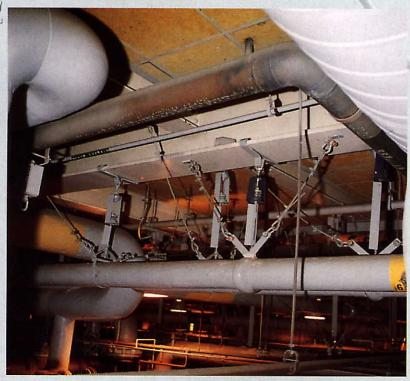
Piping with cable sway bracing survives an earthquake with no damage and no distortion. Forces in this area were high at 0.9gV and 1.2gH.
