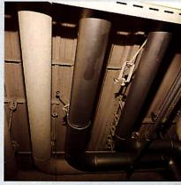
Piping without sway braces will shift position and change elevation. One hanger broke completely free and one pipe is displaced approximately 12" from its original location. On other jobsites, piping systems came down. Sway bracing and axial restraint is essential along with vertical limit stops at anchorage locations. Clevis bolts must be sleeved or braced as well.
