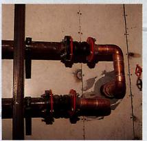
Even a very fragile copper pipeline with sweat fittings will survive at the equipment interface if proper flexible joints are used. This system was subjected to approximately 0.2gV and 0.25gH, and showed no signs of failure because of the flexibility of the twin sphere rubber connectors. (Mason Twin Sphere Superflex shown. Current improved design is Mason Safeflex.)
