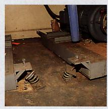
This is an excellent installation using all directional seismic snubbers to prevent the concrete bases going into resonance as would happen if the springs were used alone. There is no reason to bolt the springs to the floor as the snubbers restrict motion and the springs do not shift on their friction pads. Snubbers must always be anchored with proper anchor bolts. (Mason BMK Bases, SLF Spring Mountings, Z-1225 Snubbers)
