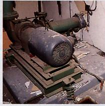
Another example showing free standing springs cannot be used without snubbing devices. The anchor bolts under these spring mountings were too close to the edge, and broke the housekeeping pad. Forces were relatively low at 0.2gV and 0.25gH, but more than sufficient to create havoc on this unsnubbed, resonant system.
