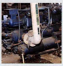
Another example of gray iron mounting failure. Fragments shown in the lower left and lower righthand corners can be dangerous to building personnel as well as equipment. Not only is the compressor out of service, but there is the additional worry of potential liability and damage.
