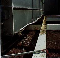
The independent rails rotated around their longitudinal axis, snapping anchor bolts
