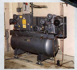
This is a simple isolation method for a horizontal tank mounted compressor (if the base legs are sturdy enough) without the use of a supplementary steel base. Mountings have built in seismic snubbers with ratings from OSHPD in the State of California. Not only these mountings, but similar designs were successful in every reviewed location. Forces were approximately 0.2gV and 9.25gH. (Mason SLRA Mountings)
