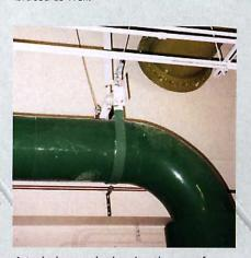
A typical example showing the use of a cable sway brace with swivel fittings for the specific purpose. Fittings are adjustable and the installation simplified by their use. (Mason Type SCB)
