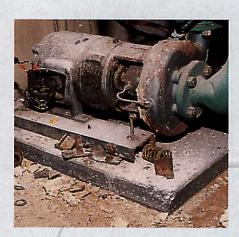
Gray cast iron spring housings invariably shatter as shown. The shrapnel flies in areas that may be occupied by plant room personnel. The only acceptable castings are ductile iron or cast steel.
