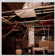
Suspended ceilings sustained damage in many installations, because sway wires were not used at all or installed improperly. Damage was extensive and very dangerous to people in the spaces below. Fortunately, the earthquake occurred when most offices were not occupied. Forces in this location were 0.2gV and 0.25gH.
