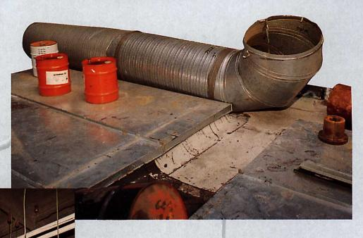
Duct work is very susceptible to seismic damage. Notice the straps that held the ducting that is now on the floor shown in Photograph to the left. This can be prevented by the use of sway bracing to limit sway and keep the duct work in place. Input was 0.15gV and 0.2gH.
