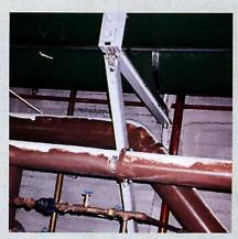
The swivel sway brace fittings at the ends of the angle iron brace eliminate welding, fitting and fabrication time. Solid sway braces can only be used on equipment that is not isolated. When equipment is isolated, bracing must be by cable or isolated devices to prevent transmission of vibration. (Mason SSB)
