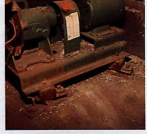
Mounting a pump directly on mountings without a supplementary steel or concrete base is bad practice because of pump coupling alignment problems when torque twists the bases. The mounting housings proved inadequate as the vertical restraining bolts failed. The restraining angles bent and either the anchor bolts were sized inadequately, of the wrong type or poorly installed as the anchorage broke free and the pump shifted out of position. Input was a low 0.2gV and 0.25gH.
