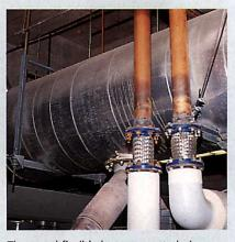
The metal flexible hose prevented pipe failure. However, the metal hose on the right was compressed. Braided metal hoses cannot accept compression and it had to be replaced. Flexible metal joints do not have the same movement capabilities as rubber joints, and tend to fail under seismic conditions. The seismic input was 0.15gV and 0.2gH. (Recommendation: Mason Safeflex SFDEJ)
